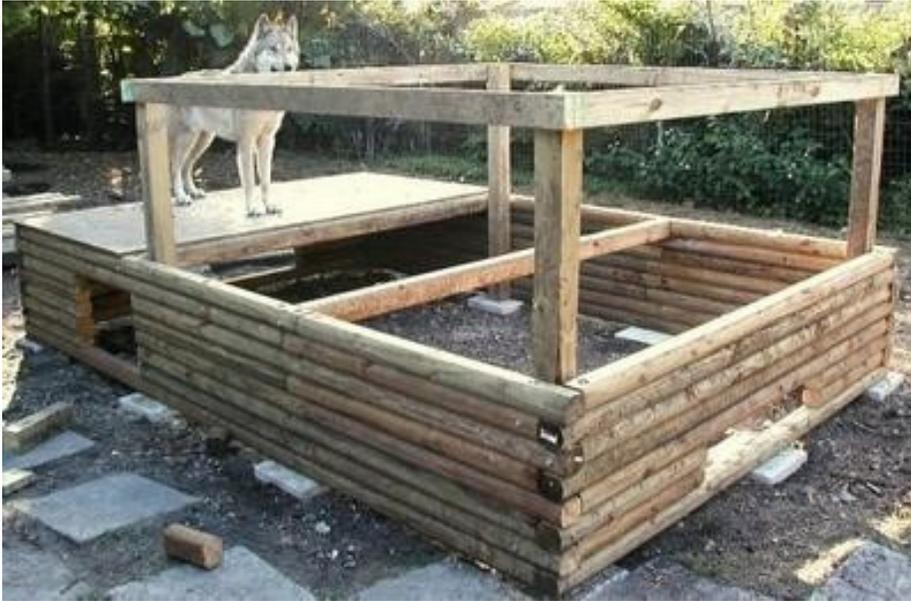
Pressure treated landscape timbers were used to build the “log cabin” exterior. The 8’x12’ decking on the first floor was created using three sheets of 3/4” pressure treated plywood, which was supported by the landscape timbers on the outside and pressure treated 4”x4” beams on the inside, with 4”x4” support cross braces (as shown in the bottom photo).
