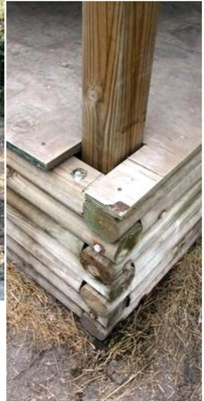
The landscape timbers are screwed together end-to-end and top-to-bottom using galvanized lag bolts. The 4”x4” uprights were attached to the timbers, also using lag bolts.
